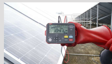
Energized device test (DC 1000V; PV)
